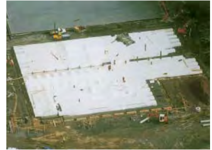
Harvey Norman Building, Whangarei
