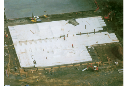
Harvey Norman Building, Whangarei
